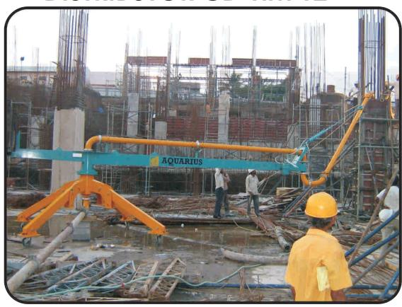
The **AQUARIUS CD-HM 12** provides an inexpensive solution, as a practical complement to stationary concrete pumps, when separate concrete placing booms cannot be used to their full value. The reach of a placing boom on a truck mounted concrete pump can also be improved with the help of this distributor in the decisive last few meters to give a more extensive working range.
